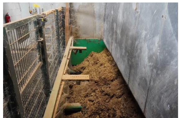
Feedstock is supplied by a screw pump.
