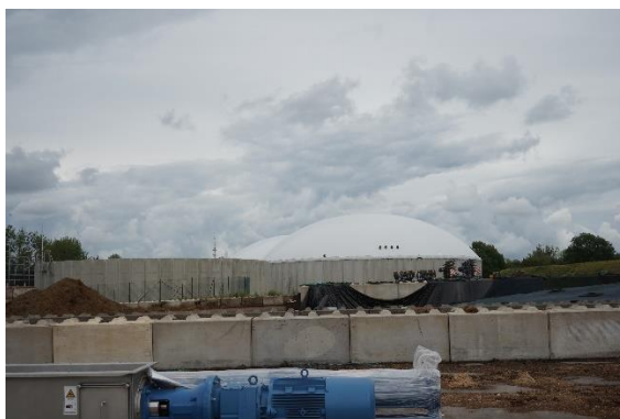
The plant is being expanded in order to produce biogas for the transportation sector.
