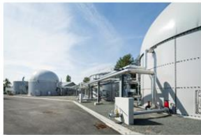
Biogas Pilot Plant 沼气厂
