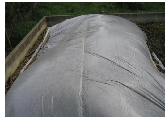
Figure 19: Gas sampling from open biofilters (Source: gewitra)
