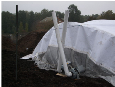
Ambient air supplied to the wind tunnel with two separately installed fans and supply air ducts (front view of the wind tunnel)
