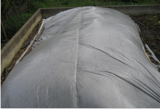
Figure 5.5-1: Gas sampling from open biofilters (Source: gewitra)
