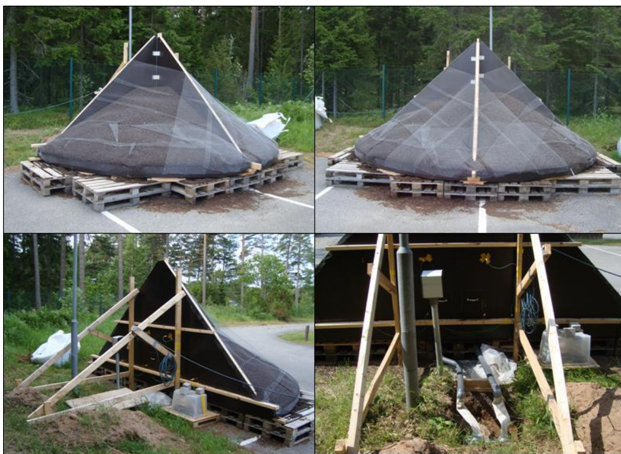
Figure 33: Outdoor storage construction used for testing of the SECTOR spruce and poplar pellets at Vattenfall's R&D centre in Älvkarleby, Sweden.
