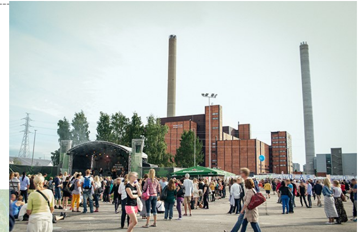
Hanasaari power plant B, nominal output 321 MW
