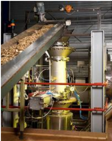
Feeding of biomass on top of the reactor
