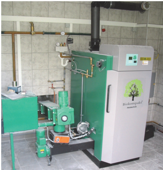
Figure 2: combustion unit - Biokompakt AWK ECO 80
