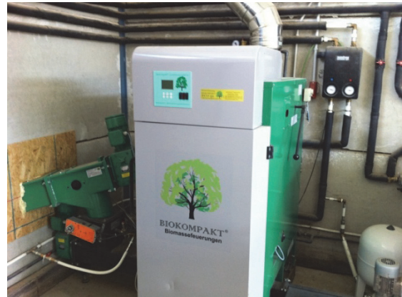
Laboratory with Biokompakt AWK boiler. An adjusted combustion technology is important.
