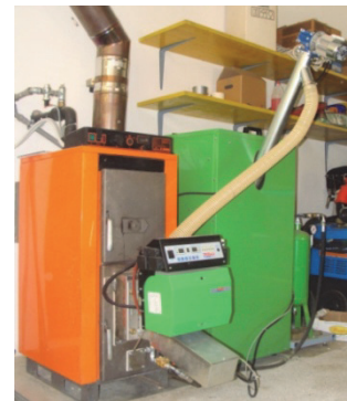
Picture 2: Termocabi burner for agri-pellets implemented in a traditional boiler for wood fuels.
