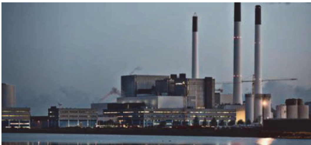
Amagerværket in Copenhagen is a very large Power Plant supporting the city with district heating and electricity. The plant is designed for both coal and biomass and has advanced flue gas cleaning systems
