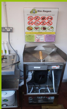
a) Bio-Regen Food waste processing machine supplied by Bio-regen Photonics
