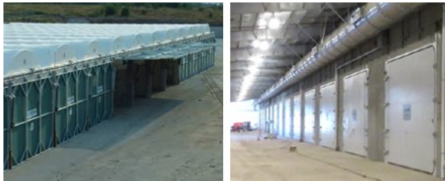
Figure 23: Different type tunnel composting installations (Eggersmann)
