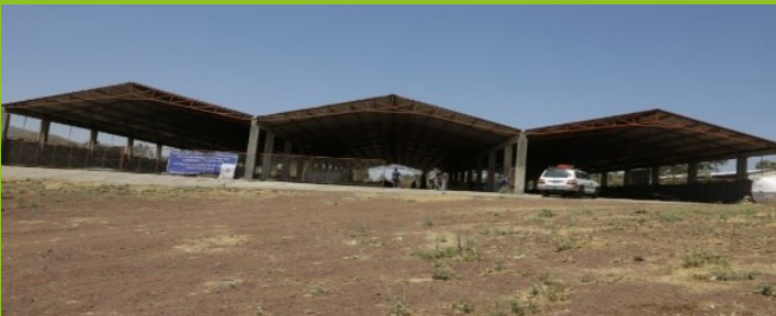
Figure 20: Compost shelter for windrow composting pilot in Bishoftu, Ethiopia [Picture and further reading source: (UNDP 2017)]
