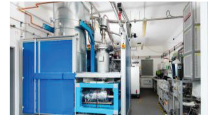
FUEL TECHNICAL CENTER
